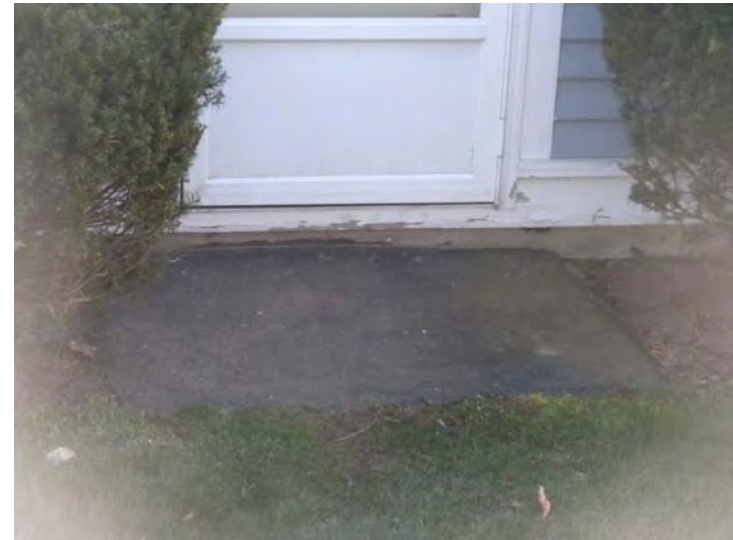
View of the rotting/deteriorating kick-plate and wood trim
