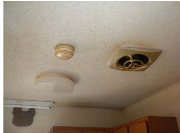
Heat sensor and exhaust fans in each kitchen
