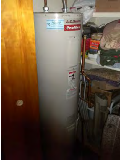
Electric domestic hot water tank
